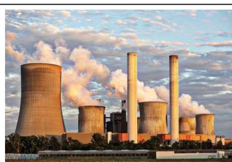
Figure 3: Cooling Towers (Alec, 2017)
