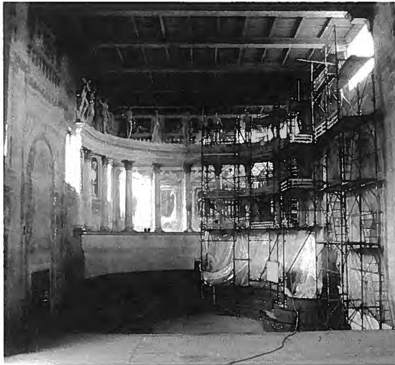
View of the loggia from the stage during partial renovation.
