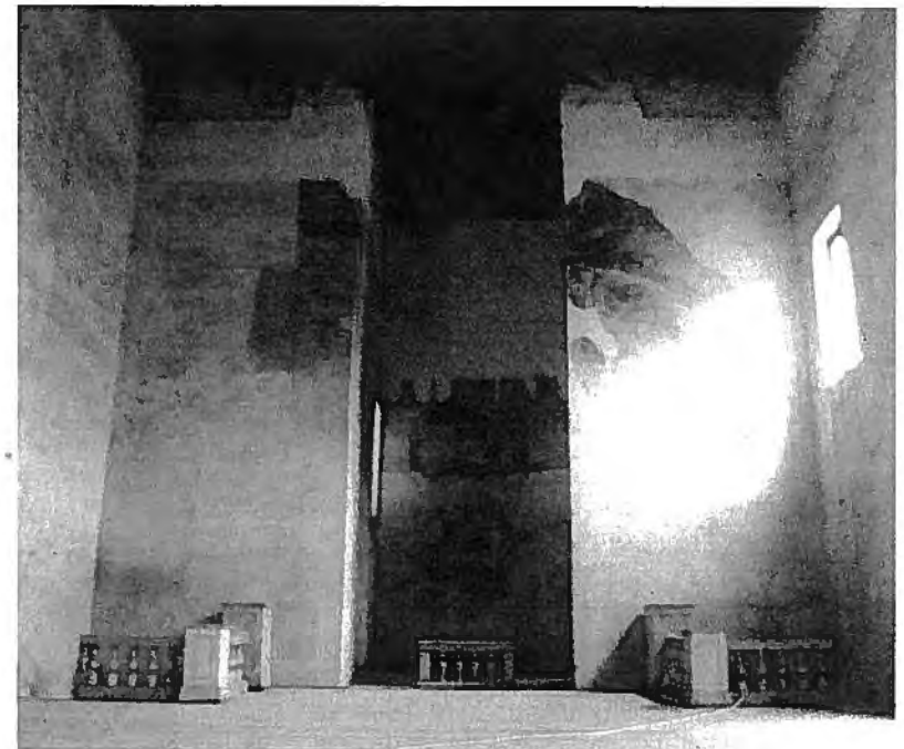
View of the performance area, showing the raked stage and fragments of frescoes thought to be background scenery.
