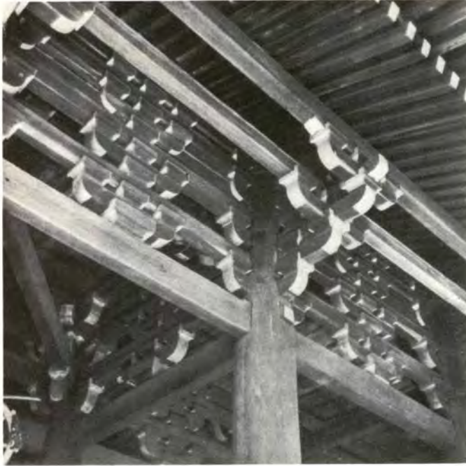
8. Bracketing of the Sammon (gate building) of the Zen temple Tofukuji, Kyoto.
