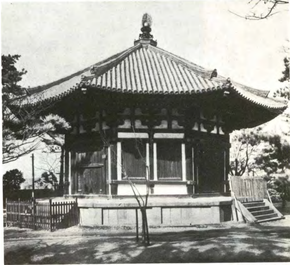
5. Northern Octagonal Chapel (Hokuen-dô) of the Kôfukuji, Nara.
