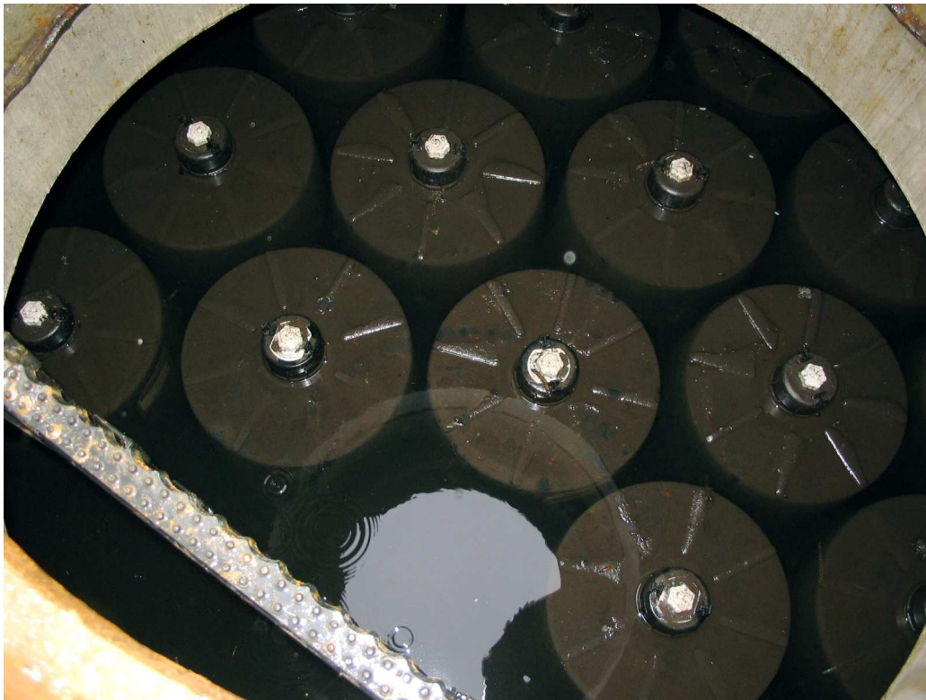
Figure A6: Photograph of the Alabama Hill vault, November 2005.
