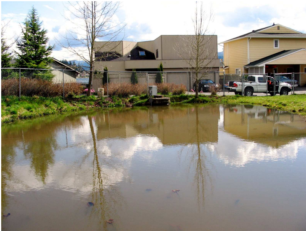
Figure A8: Photograph of the Park Place wet pond, March 2005.
