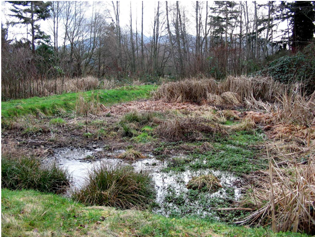
Figure A11: Photograph of the South Campus storm water treatment facility, January 2005.
