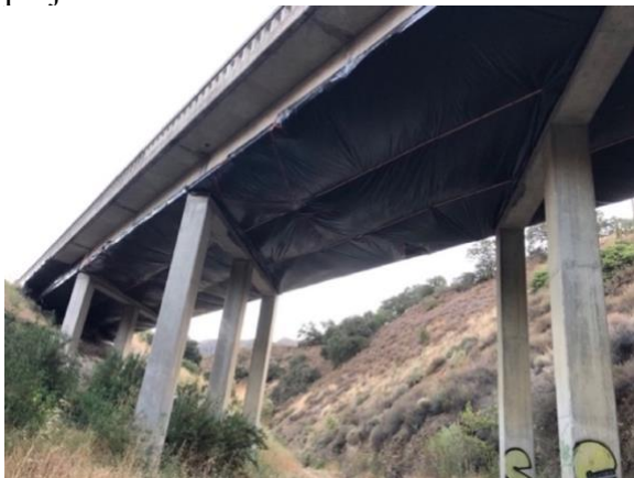
Figure 14: Image of the Northbound bridge off Highway 101 at Nojoqui Creek in Santa Barbara County showing the bat exclusion material. Image taken by Maddie Zambo on July 13, 2022.
