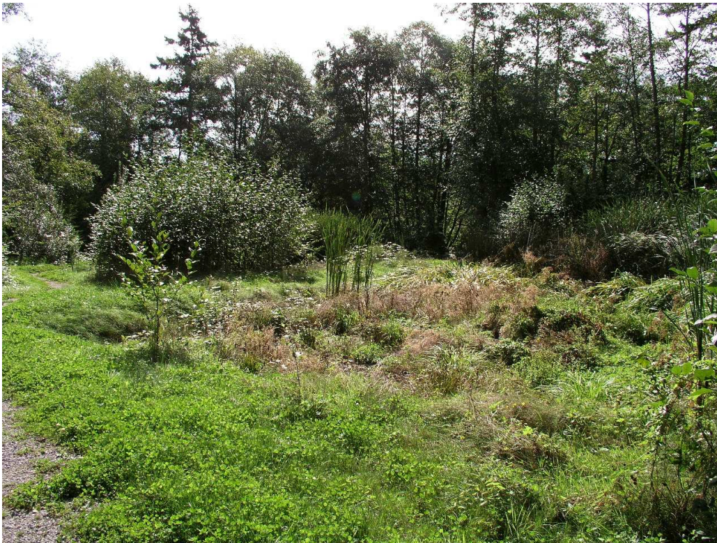
Figure 36: South Campus storm water treatment facility, August 26, 2004.
