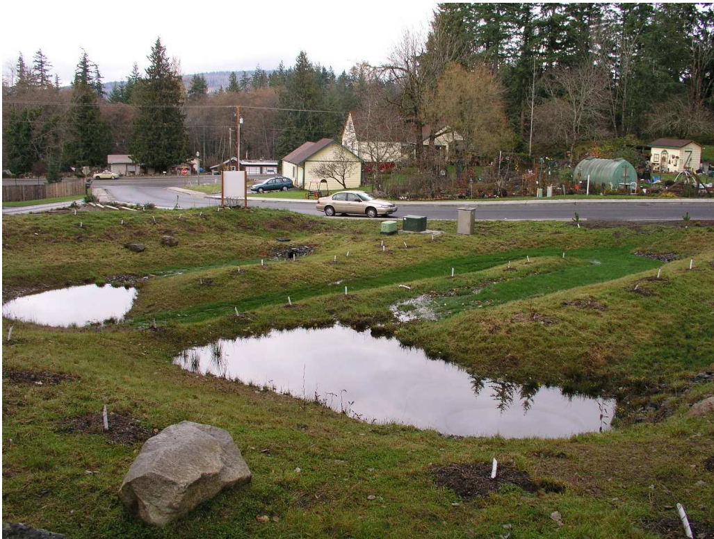
Figure 37: Parkstone water treatment facility, November 20, 2003.
