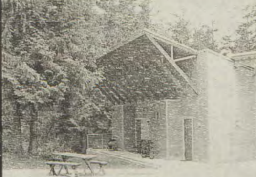
The Shannon Point Facility.
