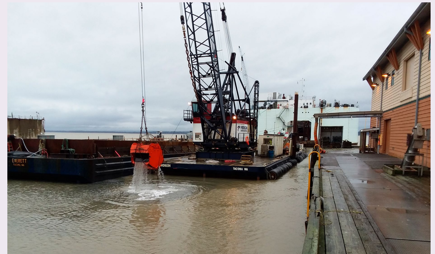
Dredging of contaminated sediment Photo: Washington State Department of Ecology
