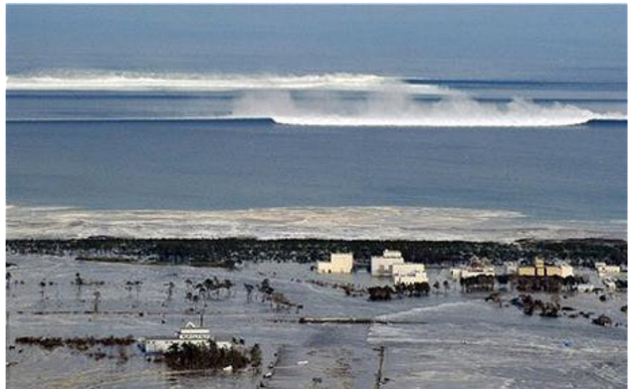
Figure 3. Following the 2011 Tohoku earthquake, multiple tsunami waves inundated Natori city, over a period of hours. Source: Reuters.
