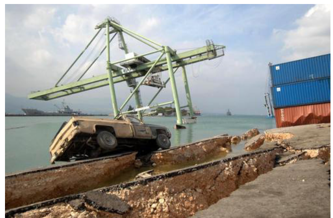
Figure 49. The 2010 M7 Haitian earthquake caused high damage to the main port terminal in Port-au-Prince. Seismically induced lateral spreading caused a shipping-container crane to tilt toward the harbor. Photo: Daniel C. Pearson, U.S. Navy.
