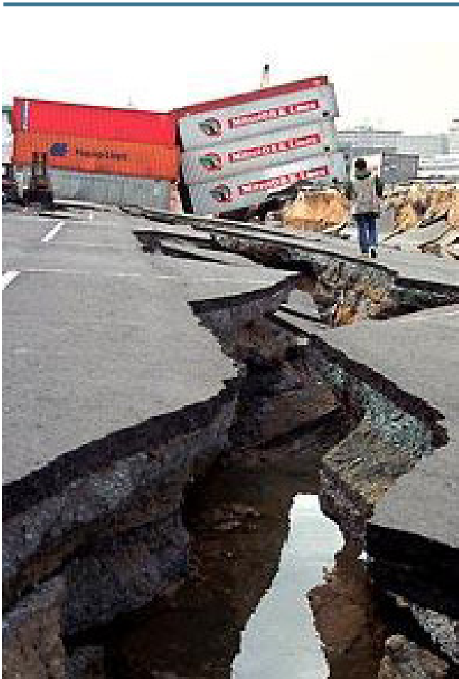
Figure 47. Liquefaction resulting from 1995 M 6.9 Kobe earthquake caused high damage to facilities at the Port of Kobe. The liquefied soil pushed against a major retaining wall causing it to slide five to ten feet toward the water. This movement caused settlement of the retained soils and destroyed structures supported by these soils. Photo: Koji Sasahara, AP.
