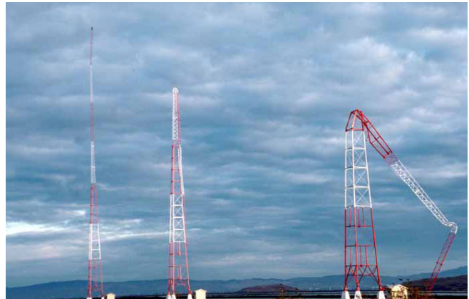
Figure 105. Shaking from the 1989 M6.9 Loma Prieta earthquake damaged radio transmission towers in California. Even radio and cell towers that do not experience severe damage may still be un-operational after the quake if antennae, cables, or other hardware become unaligned or damaged. Photo: USGS.
