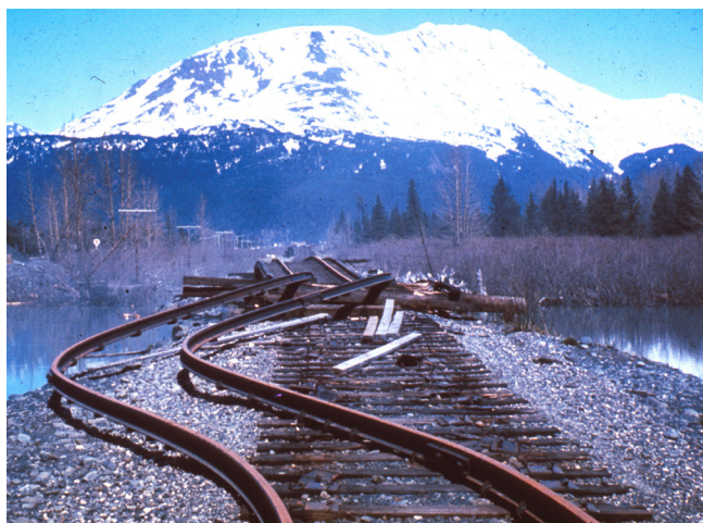
Figure 44. The M9.2 Great Alaska Earthquake of 1964 damaged extended lengths of track due to ground failure as a result of lateral displacement. This type of ground failure can tear rails from their ties and caused them to buckle. Photo: USGS.
