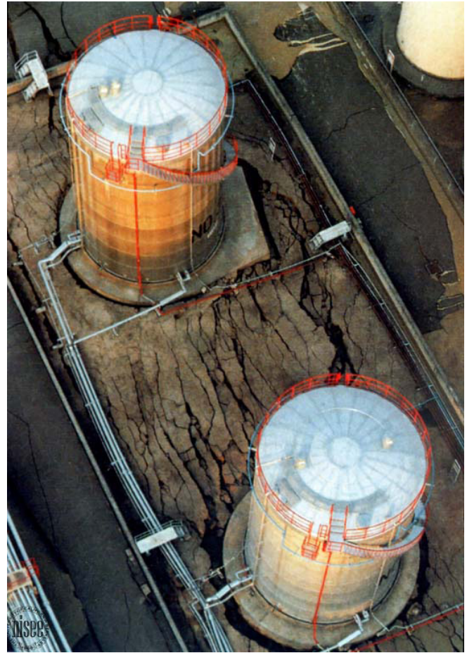
Figure 51. The 1996 M6.6 Kobe earthquake in Japan caused damage to pavement supporting tanks and other facilities. Some of Washington and Oregon's port fuel facilities, such as fuel tanks and terminals, are situated on liquefiable soil. These facilities could spill or rupture during the earthquake, posing serious fire and explosion threats. Photo: HITRAC.
