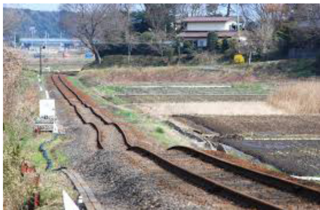
Figure 43. The 2011 M 9 Tohoku earthquake caused considerable bending of the Hitachinaka Railway tracks. Photo: Toshinoei Baba.
