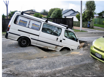
Figure 6. The 2011 Canterbury earthquake in New Zealand caused the loose sand and silt supporting the paved surfaces to liquefy and lose its ability to support this automobile. Liquefaction often results in uneven patterns of ground settlement. Photo: Martin Luff.
