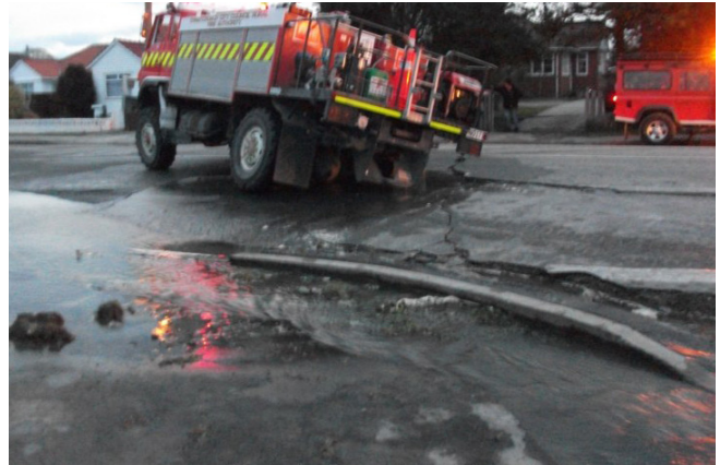
Figure 66. Liquefaction from the 2011 M6.3 earthquake in Christchurch, New Zealand trapped a fire engine in silt. Unnavigable road conditions could hinder emergency response efforts throughout Washington and Oregon.
