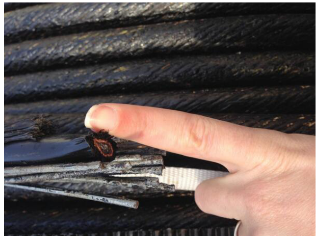
Figure 107. Internet and phone providers believe that a small earthquake severed this underwater cable and caused a phone and data outage in the San Juan Islands. Following an earthquake survivors may not be able to use undamaged landlines as the volume of emergency calls will likely overwhelm surviving infrastructure capabilities. Photo: KING.
