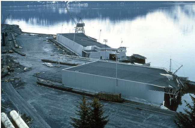
Figure 50. A tsunami resulting from the 1965 M9.2 earthquake in Alaska caused significant damage to facilities at Seward Port. In addition to infrastructure damage, tsunami currents could drastically modify the underwater topography near ports, making it difficult or even impossible for vessels to navigate. Photo: Mildred Kirkpatrick.
