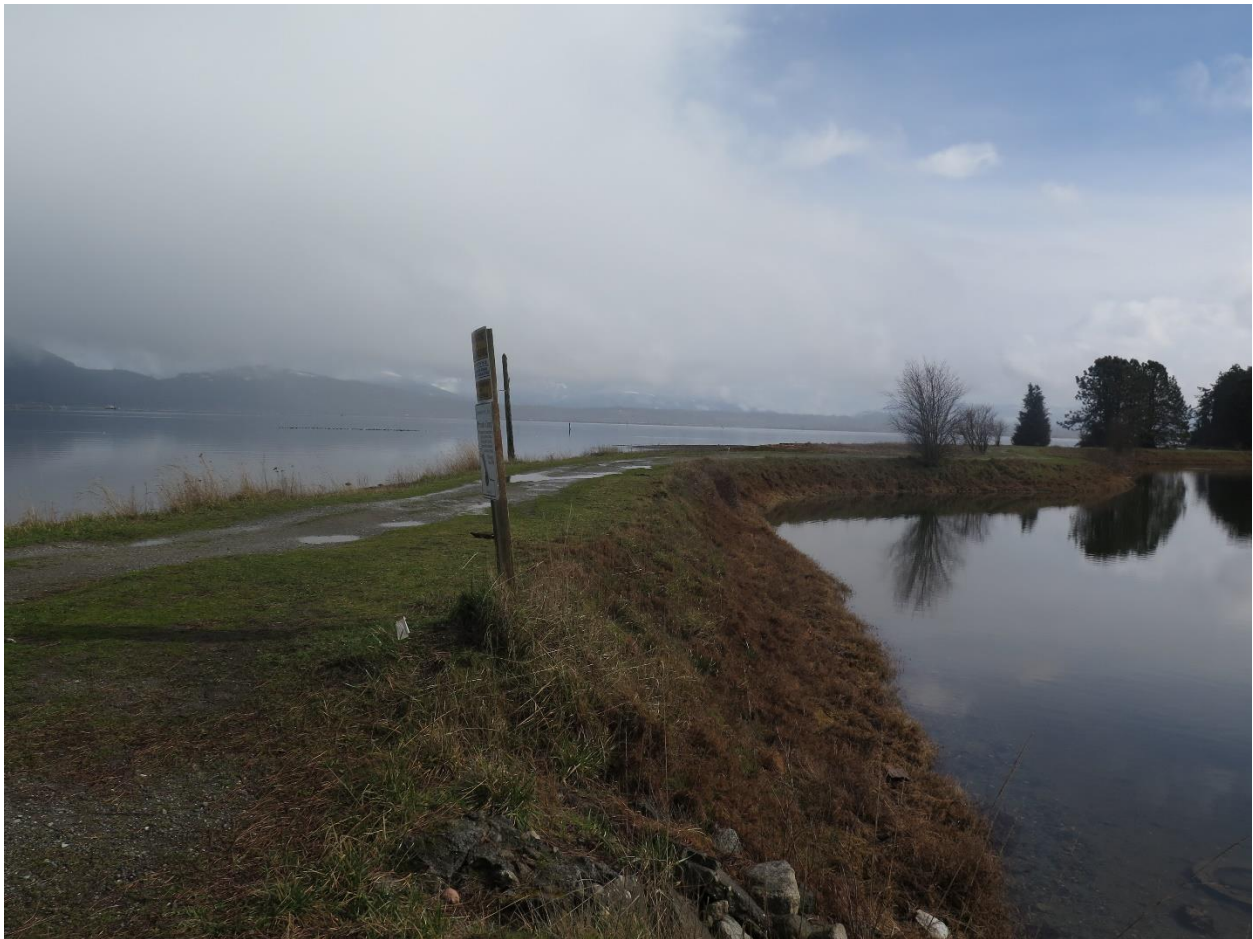
Figure 2. A photo of the dike that was constructed to create Freestad Lake. The existing estuary is on the left, and the lake is on the right, photo by Amanda Smith.
