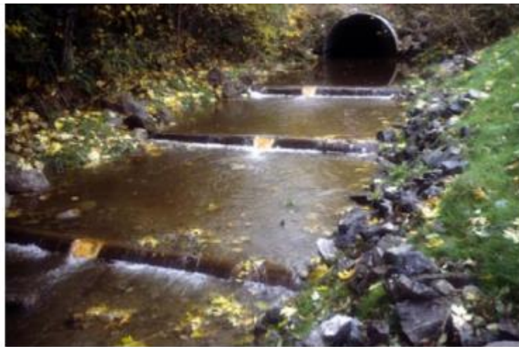
Figure 4. Example of a streambed control fish passageway, using downstream log controls to backwater a culvert (WDFW, 2009).
