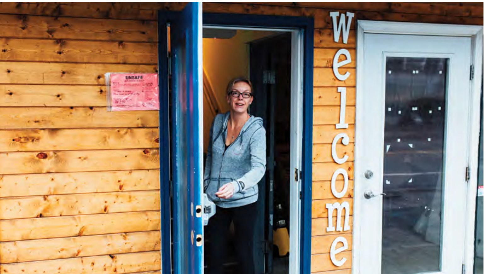
ABOVE: Jessica Pangilinan opens a door into the Bay Breeze Restaurant and Bar which was damaged after a December 2018 storm. The restaurant has been closed down since then to repair the damage and all employees have been out of work.
