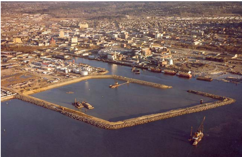
Figure 1. Construction of the ASB (Source: POB Powerpoint, 2018)
