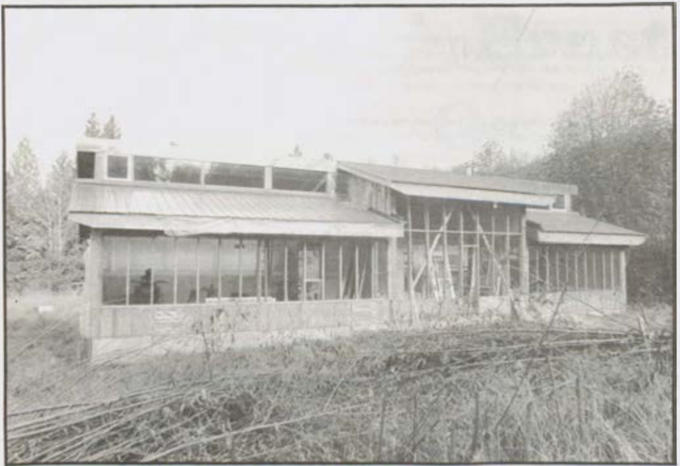
Ernst Gayden's owner-built solar home nears completion.
