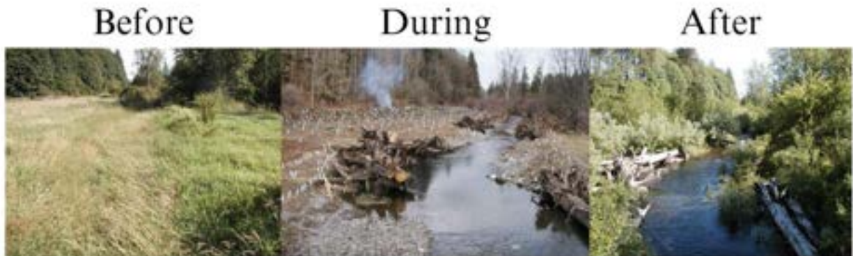
Figure 1. This diagram depicts the changes to Kendall Creek through restoration work using pictures taken by the NSEA Restoration Team. This work began in 2003 to clear the grass and create a complex habitat that salmon can utilize. The “After” picture was taken five years later, in 2008, when native plants were fully flourishing within the riparian zone.
