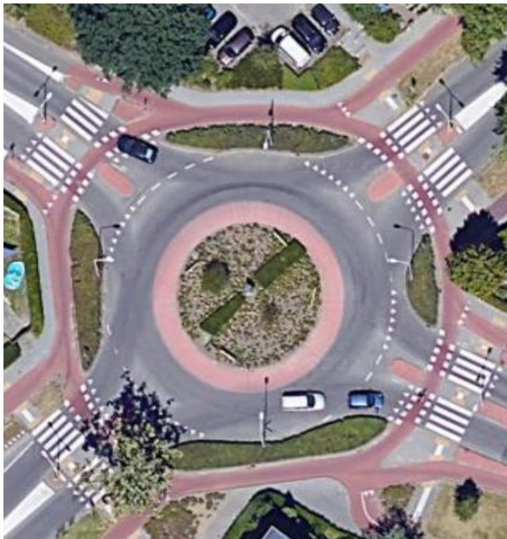
Roundabout in Nijmegen, Netherlands, with cycle tracks squished to fit its surroundings (Google Earth)
