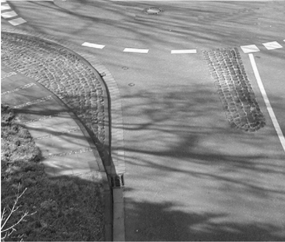
An example of use of aprons to narrow an entrance in Germany (Road and Transportation Research Association Road Design Work Group)
