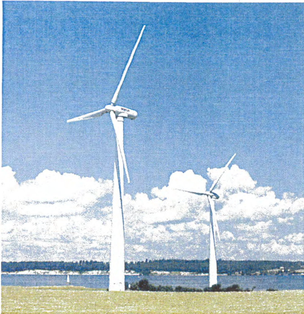
Two BONUS 450 kW wind turbines at Kegnæs Ende, Sydals, Denmark
