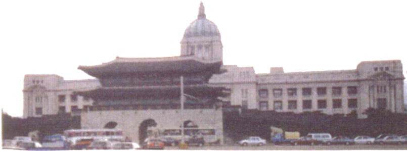
The Building preparing for demolition in 1995.
