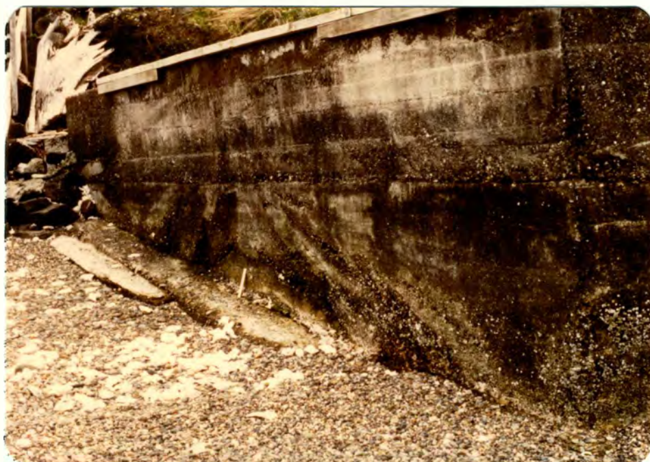
FIGURE 20: Sediment accumulated at the updrift side of a bulkhead built across the upper foreshore, along Hood Canal. Compare with Figure 21, the downdrift side of the same bulkhead.
