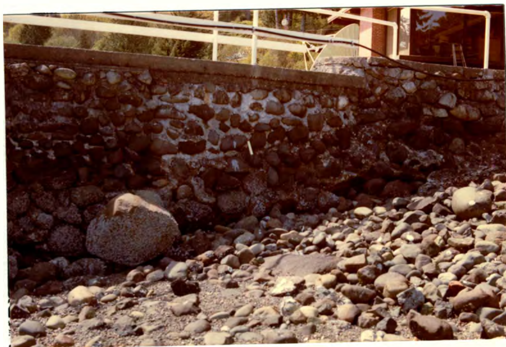
FIGURE 25: Compare the sediment size and beach level shown in this photo of downdrift side of groin to that of updrift side in Figure 24.
