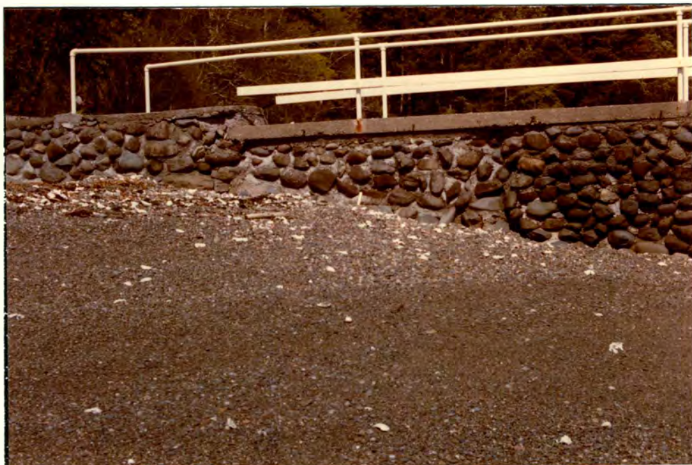
FIGURE 24: This large groin at Mike's Resort, on Hood Canal, blocks shore drift and causes sediment accumulation. Downdrift side of groin is shown below in Figure 25.
