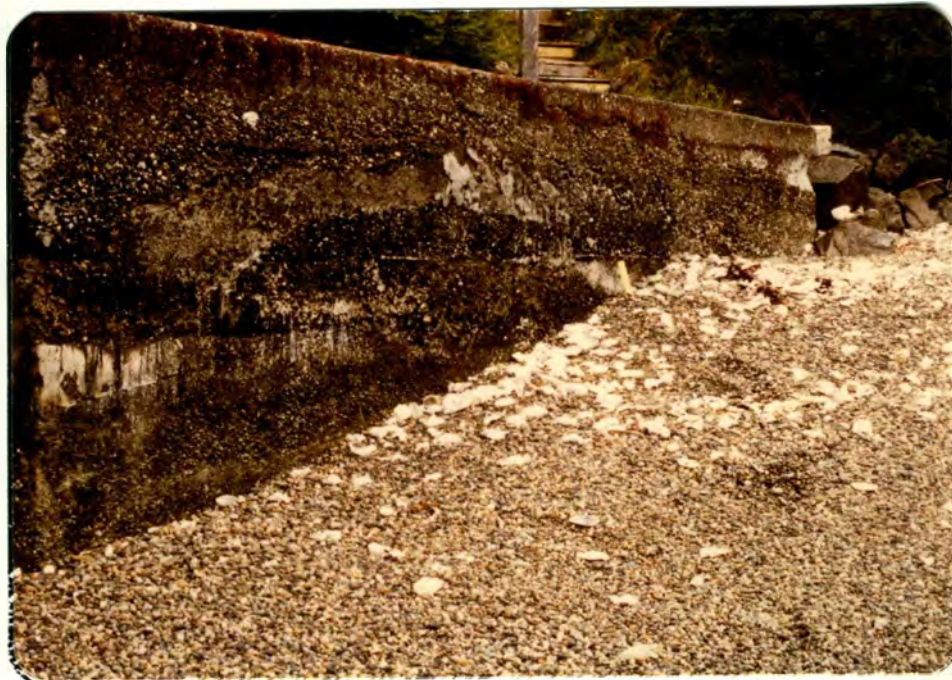
FIGURE 20: Sediment accumulated at the updrift side of a bulkhead built across the upper foreshore, along Hood Canal. Compare with Figure 21, the downdrift side of the same bulkhead.
