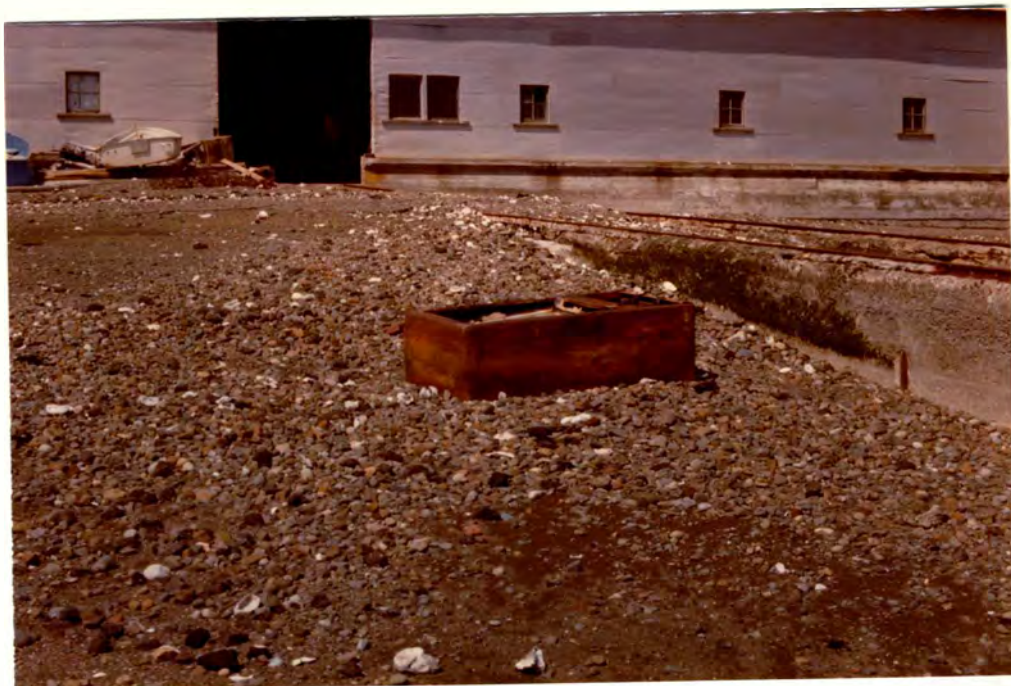
FIGURE 33: Sediment accumulated updrift (southwest) of boat ramp at Beacon Pt., Hood Canal. Note position of white boat relative to beach and compare with Figure 34.
