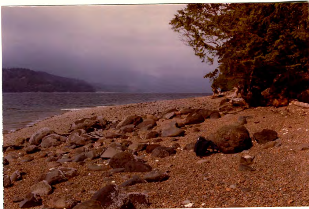
FIGURE 39: Boulders, which have eroded from the bluff along the eastern shore of Hood Canal, impede north-easterly net shore drift (note pebbly sediment to right) and protect the base of the bluff from further wave erosion.
