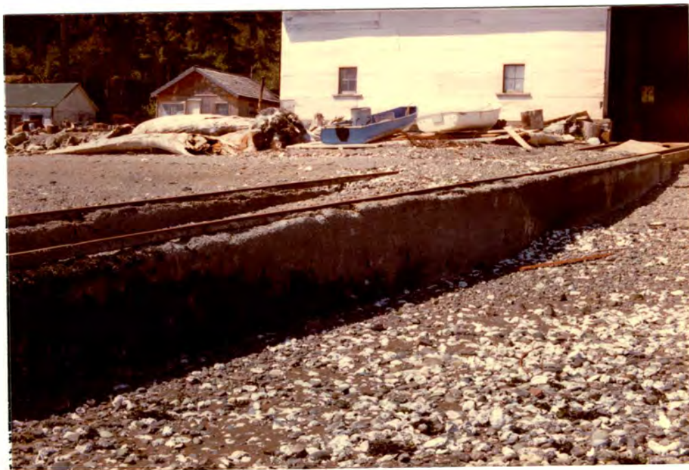
FIGURE 33: Sediment accumulated updrift (southwest) of boat ramp at Beacon Pt., Hood Canal. Note position of white boat relative to beach and compare with Figure 34.
