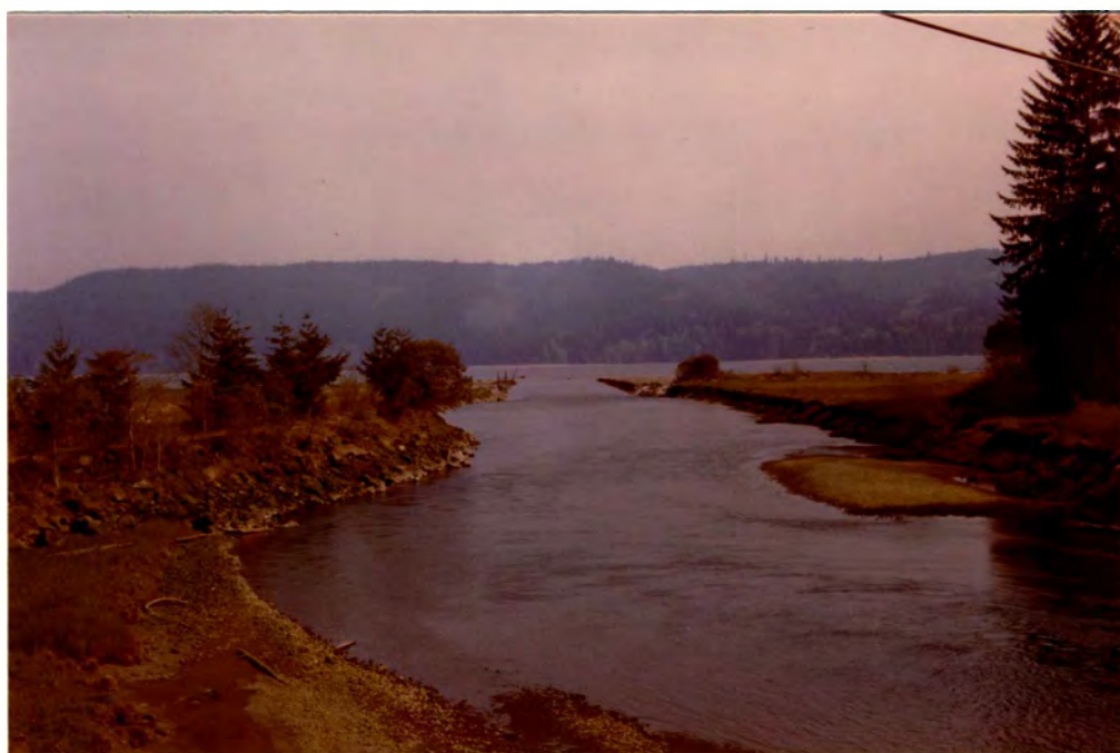
FIGURE 36: The artificial channel of the Hamma Hamma River truncates the spit which originally diverted the stream northward. Stone jetties in the distance cross the intertidal portion of the delta. View to the east.
