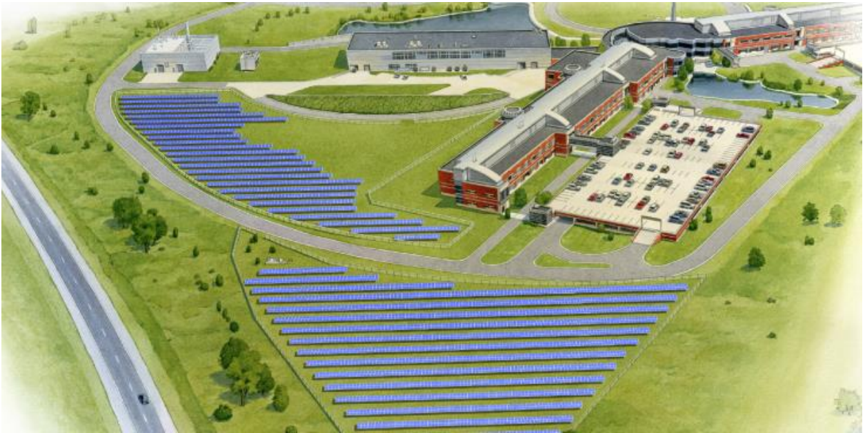
Figure 6. Community Solar Array at Western Michigan University 15
