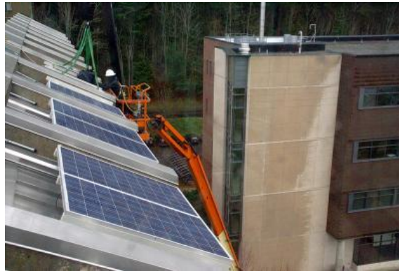
Figure 2. Installation of the Environmental Studies Solar Array 5
