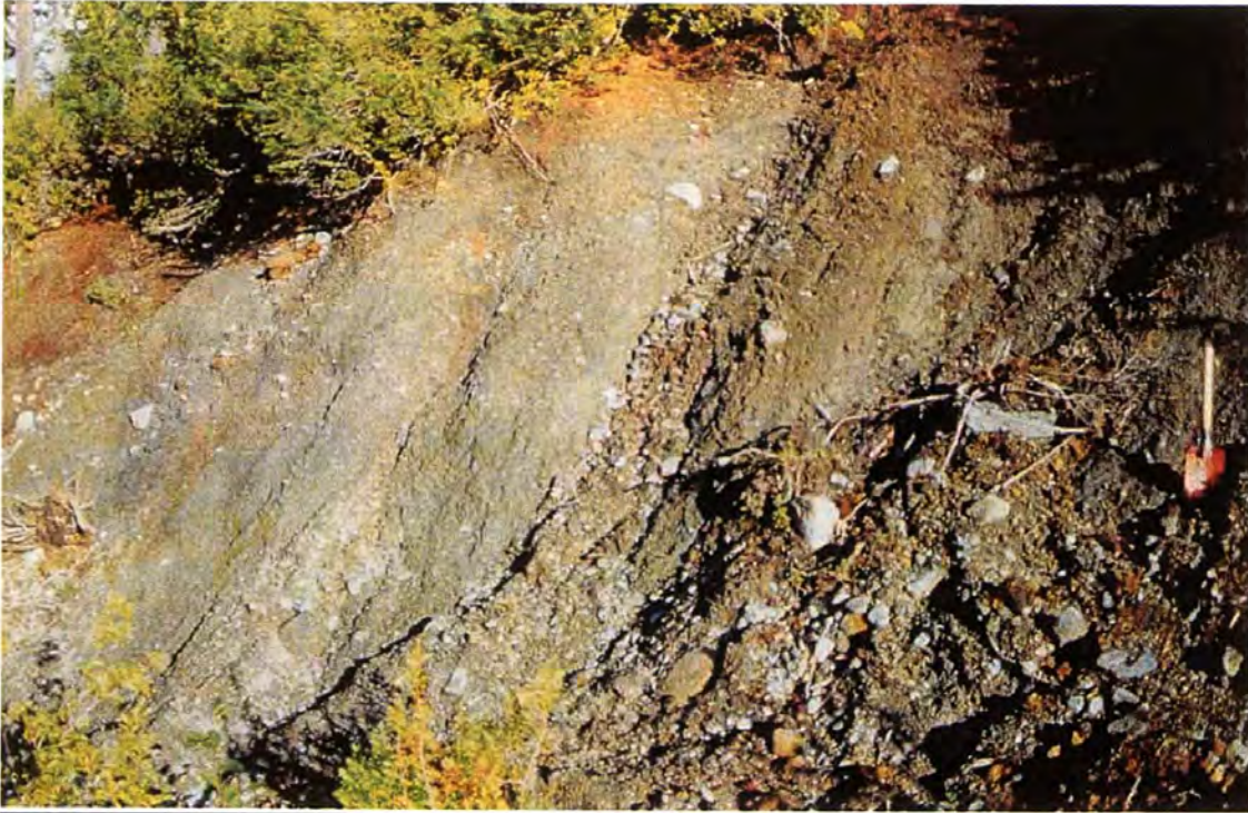
Figure 4.10 A road cut of till at the hairpin curve. Shovel on the right is ~0.5 m in height.
