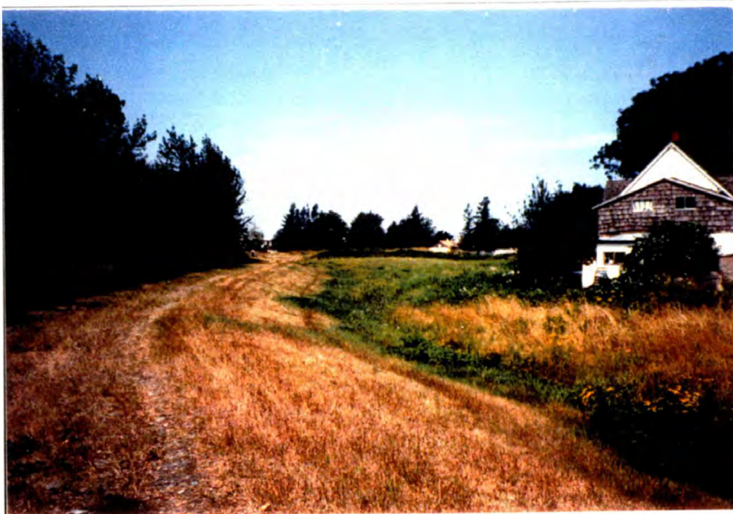
FIGURE 16: Everson Levee Extension at Everson (looking northwest). Project constructed 1991.
