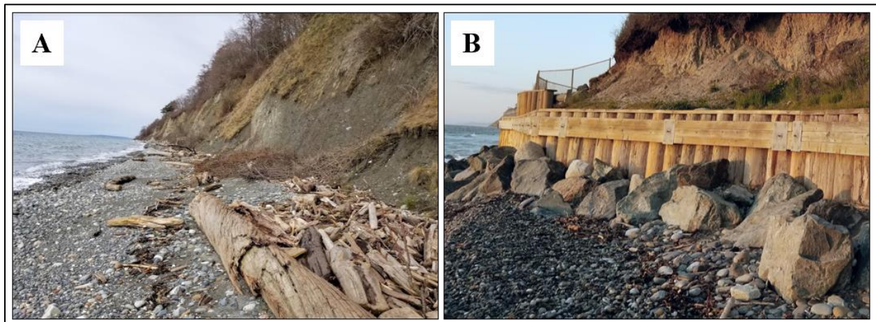
Figure 1. Photos of two typical bluff-backed beaches in the Salish Sea. Point Whitehorn Park along the Point Whitehorn Marine Reserve (A) is an example of unarmored shoreline with naturally recruited woody debris and a location on the west shore of Whidbey Island (B) is an example of shoreline armoring which includes a wooden seawall and riprap at the base of the bluff (photos by author).
