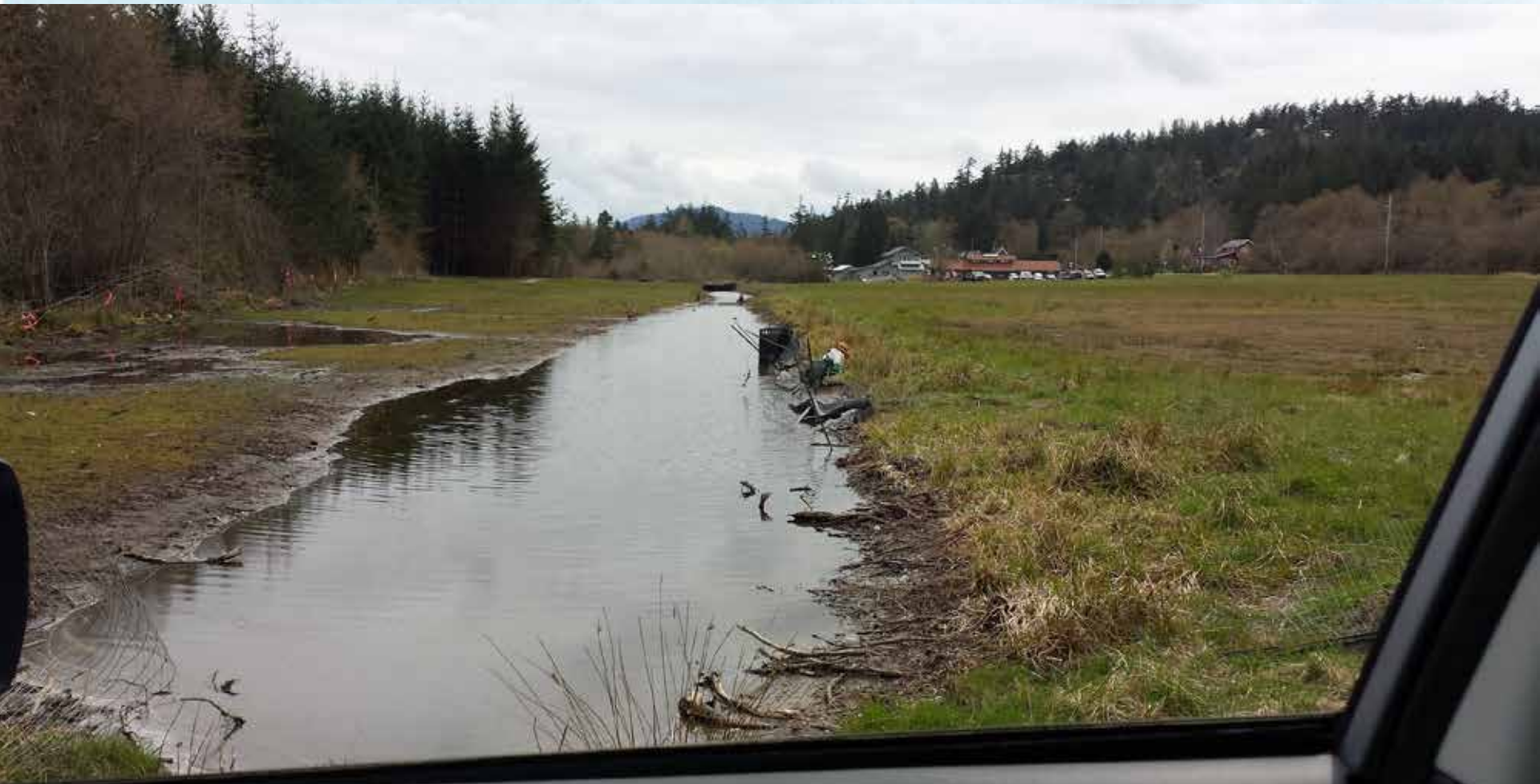
Wetland clearing and grading
