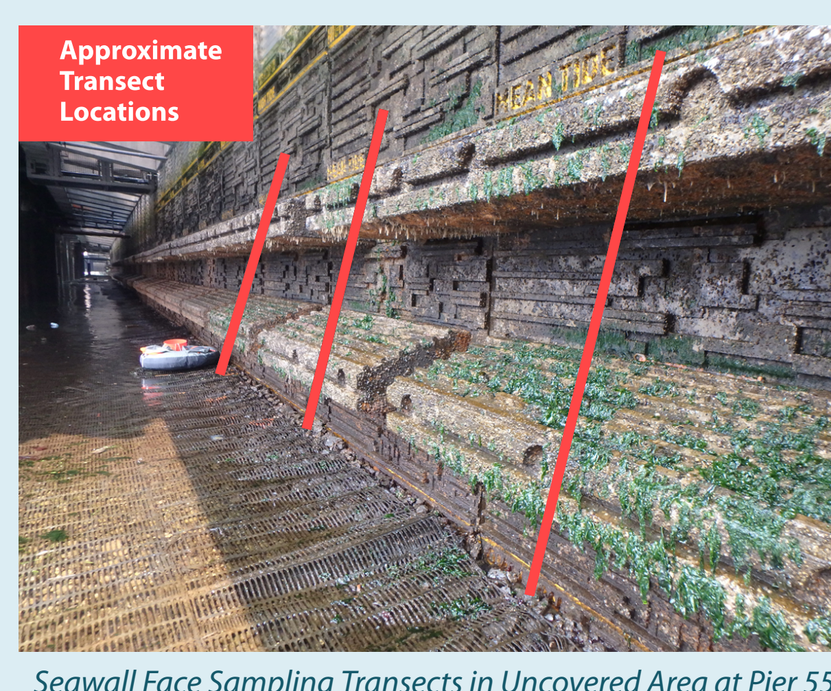
Seawall Face Sampling Transects in Uncovered Area at Pier 55
