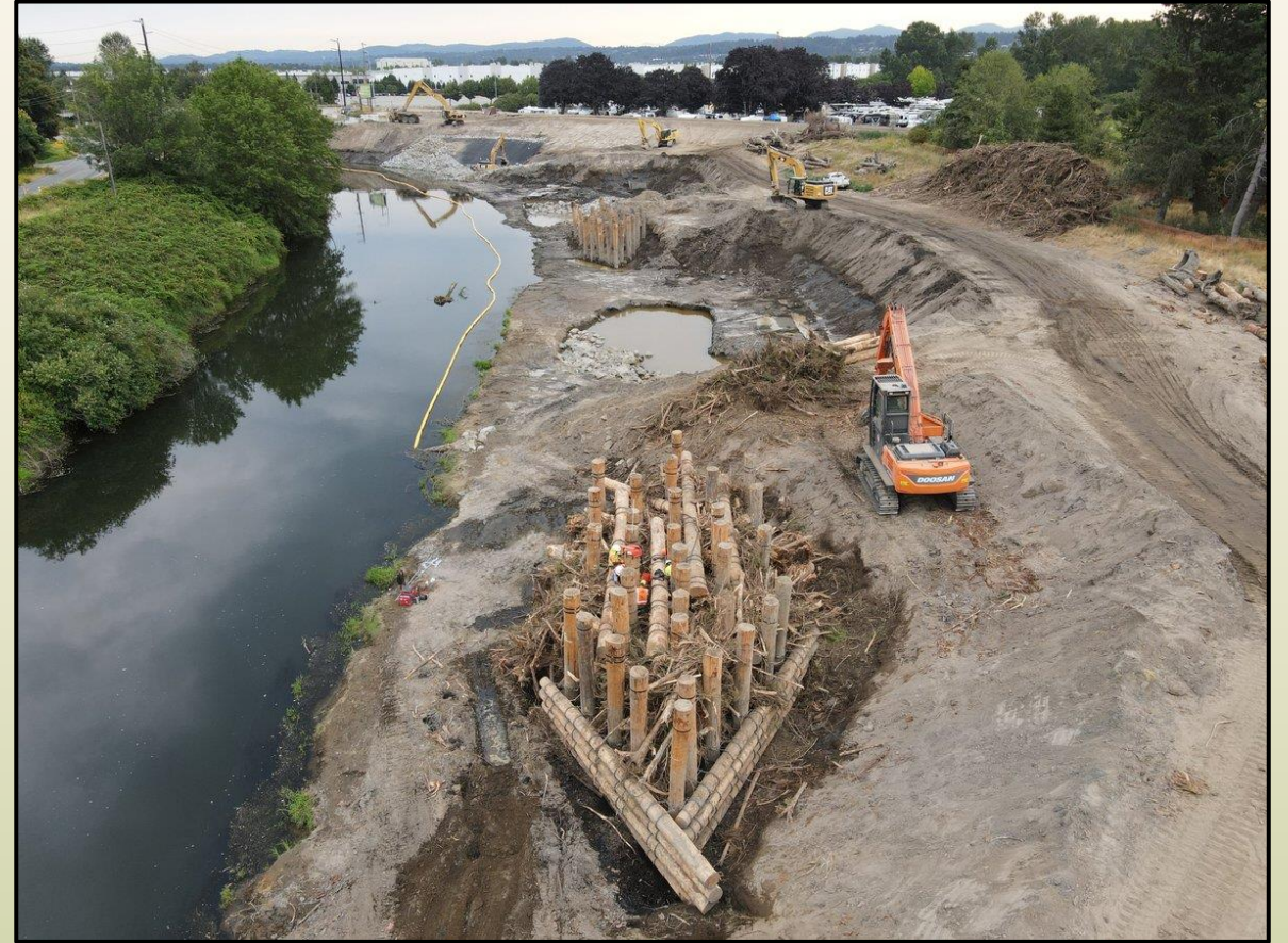
Lower Russel Construction in 2021
